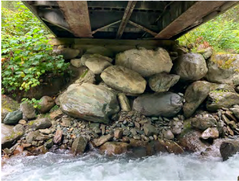
Right Bank Abutment when facing downstream
