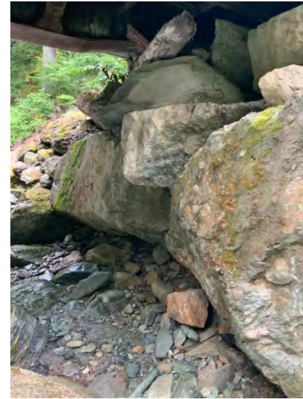
Left Bank Abutment when facing downstream
