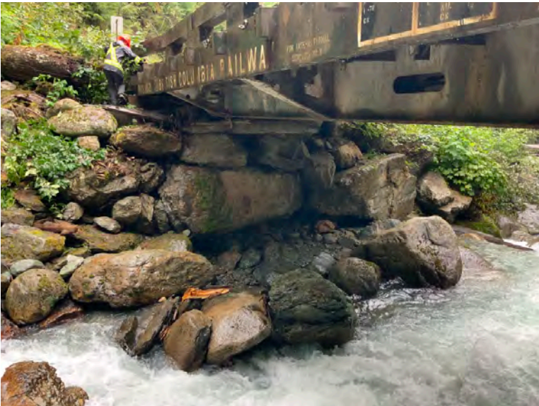
Left Bank Abutment when facing downstream
